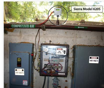
pressure is measured downstream at 110 psi, there is almost 8 percent error, which looks like a leak. Even though temperature has a smaller effect on these types of instruments, a 10 degree F change in temperature will still lead to a two percent error.
